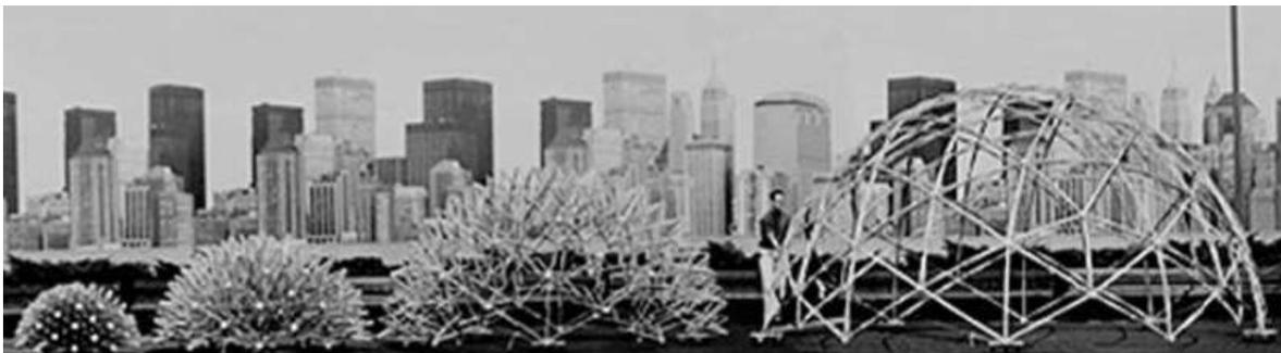
Figure 4-7: Expandable Structure, example 3, Hoberman principle.
