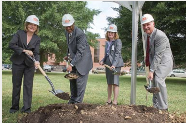
From left, Langley Director Lesa Roe hefts a shovel alongside Charles Scales, NASA associate administrator; Molly Ward, Hampton mayor; and Rob Newell, GSA regional commissioner of Public Buildings Service.
