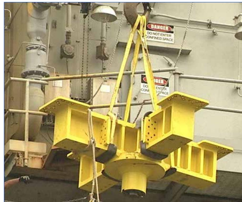
A new thrust frame adapter is hoisted onto the A-1 Test Stand late in 2013. The 7,700-pound frame is a critical component needed to anchor a rocket engine in place to allow for testing and collection of performance data.
