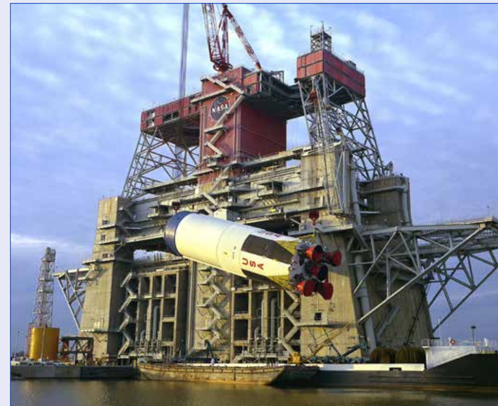
Saturn V rocket stage S-IC-9 is lifted onto the B-2 Test Stand for test firing on Jan. 10, 1969. In its early years of operation, Stennis tested the large rocket stages that powered the Apollo Program and carried humans to the moon.
