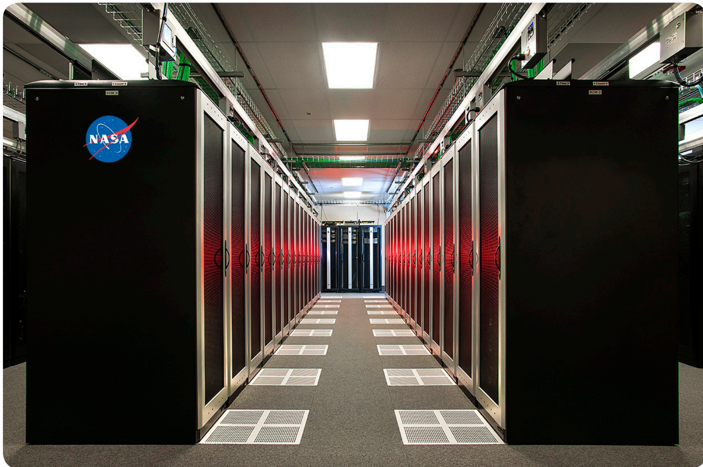
Consolidated Information Technology Center, Armstrong Flight Research Center (AFRC). Credit: Tom Tschida
