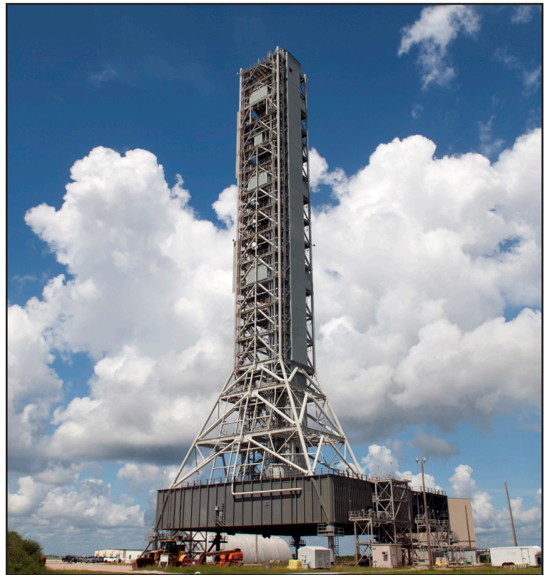
The mobile launcher that will support NASA's Space Launch System and Orion spacecraft for Exploration Mission-1 is in view at the Mobile Launcher Park Site at Kennedy Space Center. Photo credit: NASA/Cory Huston
