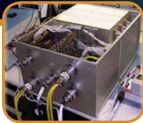
Electrical Fabrication and Assembly
