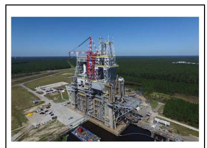
The B2 Test Stand at Stennis Space Center. This South East aspect shows the additional superstructure added to the stand to accommodate the height of the SLS Core Stage, as well as the completed tarmac in front of the stand. Exploration CoF provides construction required to support SLS, Orion, and Exploration Ground Systems program activities. Funds required for the planning and design of out-year programmatic construction remain in the applicable program accounts.
