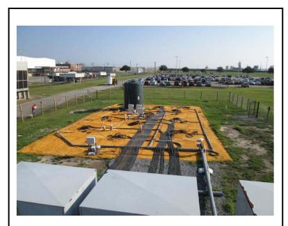
Remediation of contamination in the groundwater at MAF. Electrical current is applied through electrodes driven into the ground and the contaminated soils and groundwater are heated. The volatilized contaminants are removed through vacuum extraction.
