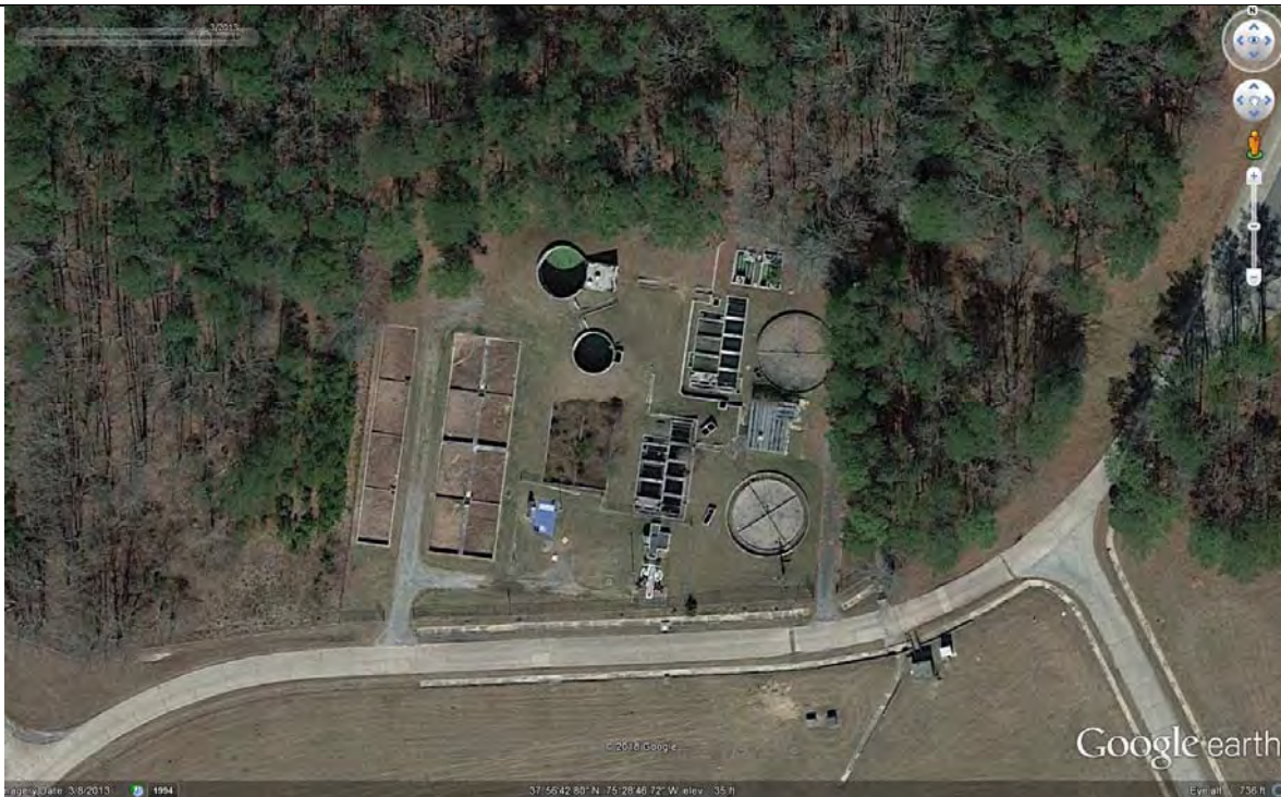
Photo: 5 | Area 5: Former Wastewater Treatment Plant
