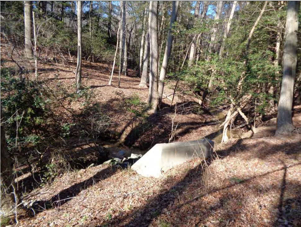
Photo: 8 | Area 8 – Wastewater Treatment Plant
