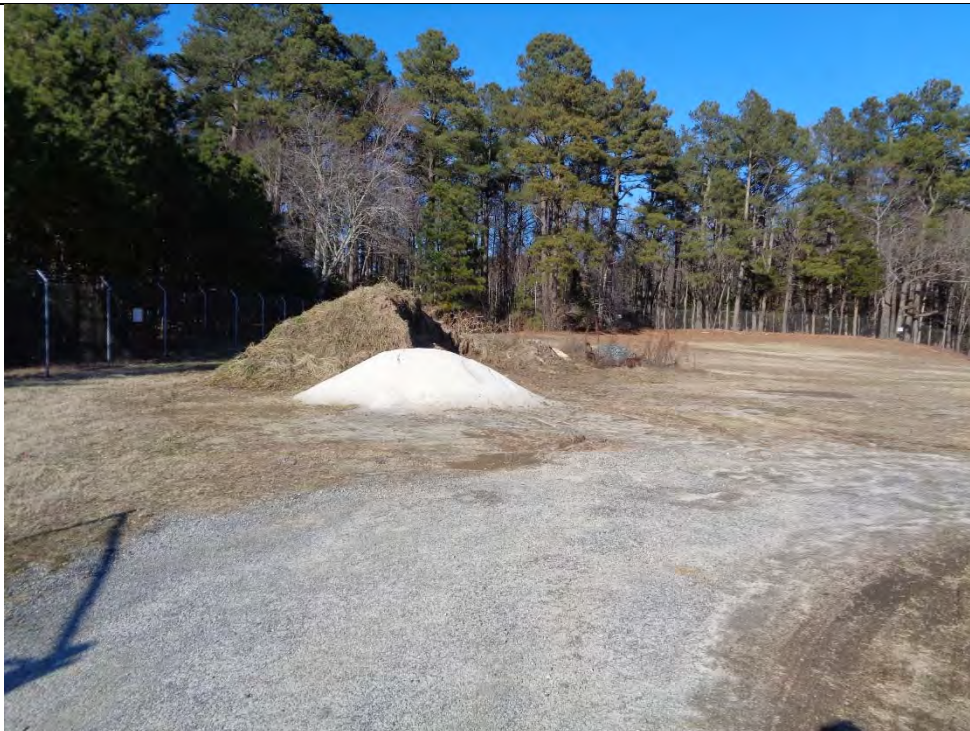
Photo: 6 | Area 5: Former Wastewater Treatment Plant
