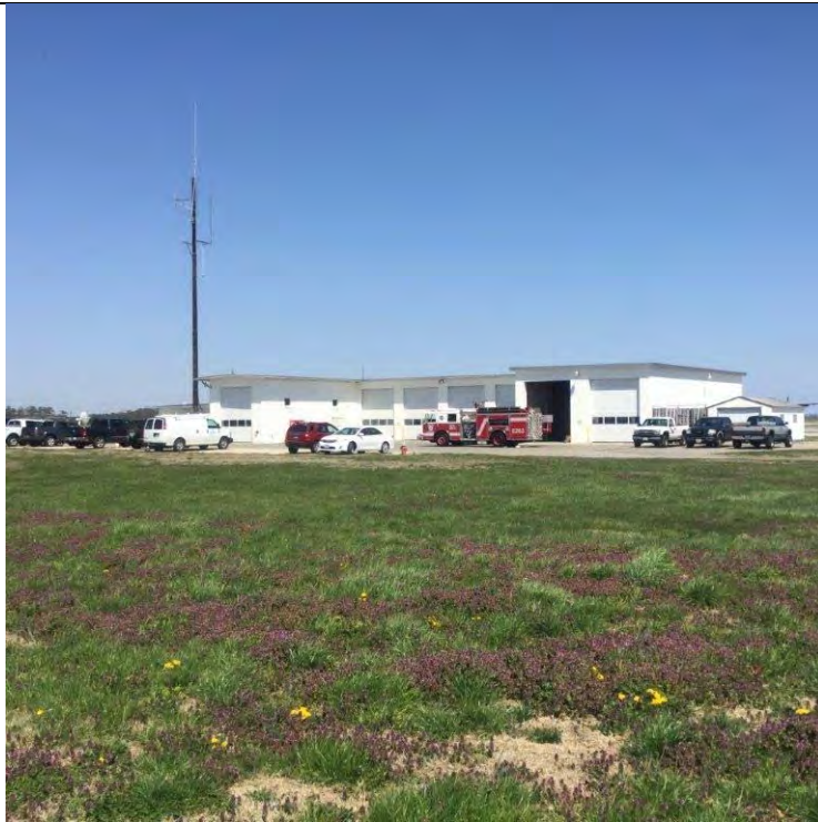
Photo: 1 | Area 1: Building B-129 Fire Station
