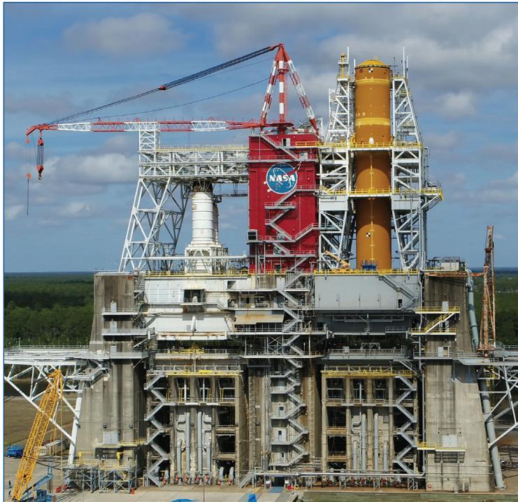
A drone image shows NASA's Space Launch System (SLS) core stage installed on the B-2 Test Stand at Stennis, where it is undergoing Green Run testing.
