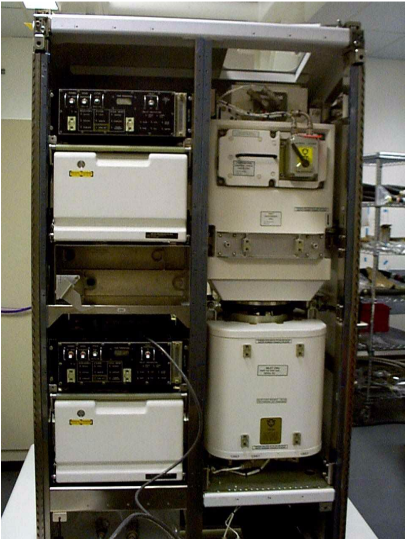
FIGURE A-4 – METOX REGENERATORS IN THE RACK
