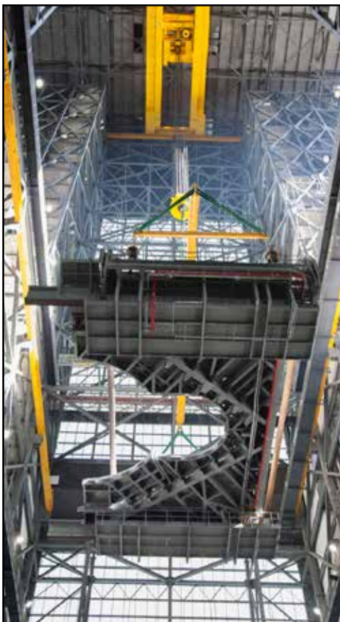
A heavy-lift crane lifts the first half of the F-level work platforms, F south, for NASA's Space Launch System (SLS) rocket, from the floor of the Vehicle Assembly Building (VAB) at Kennedy Space Center on July 15. Photo credit: NASA/Bill White
