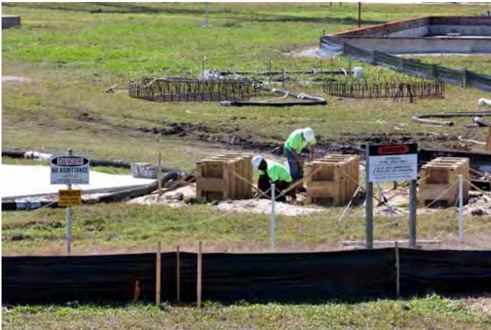
Construction workers stage parts and equipment for a new liquid hydrogen storage tank nearby Launch Pad 39B at NASA's Kennedy Space Center on February 22, 2019. The tank will support fueling of the agency's Space Launch System rocket. Photo credit: NASA/Kim Shiflett
