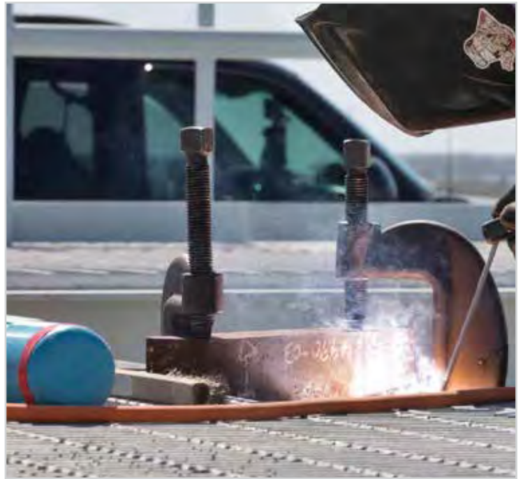
Upgrades Continue at Launch Complex 39B
