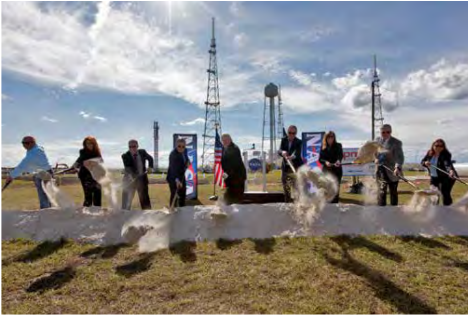
Agency and contractor managers break ground for a new liquid hydrogen tank on December 19, 2018, at Launch Complex 39B at NASA Kennedy Space Center. The storage facility will hold 1.25 million gallons of the propellant for NASA's Space Launch System rocket designed to boost the agency's Orion spacecraft, sending humans to distant destinations such as the Moon and Mars. Photo credit: NASA/Kim Shiflett
