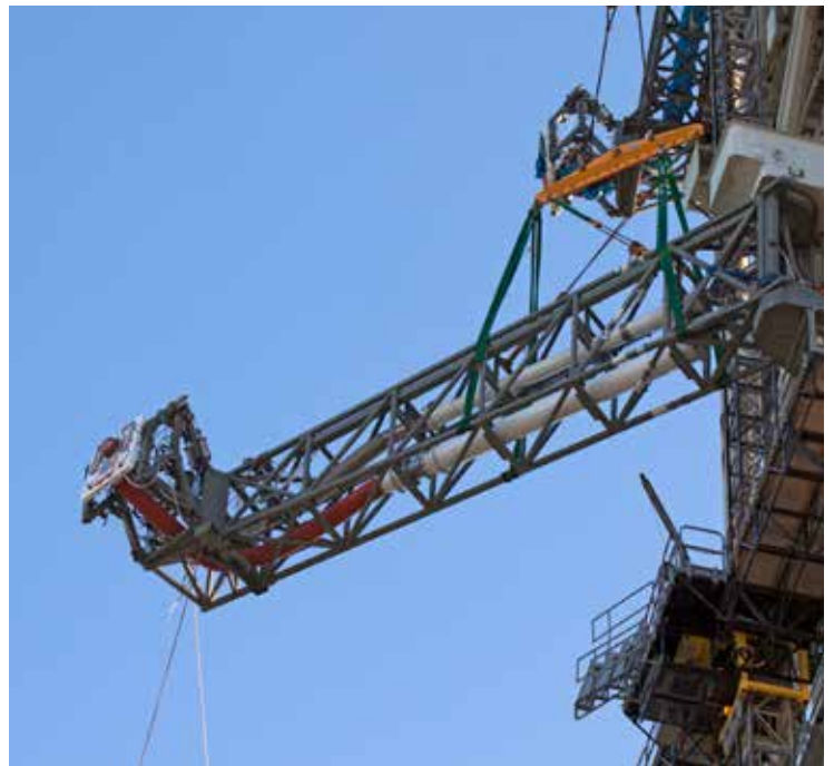
23 Core Stage Inter-tank Umbilical Fit Checked on Mobile Launcher
