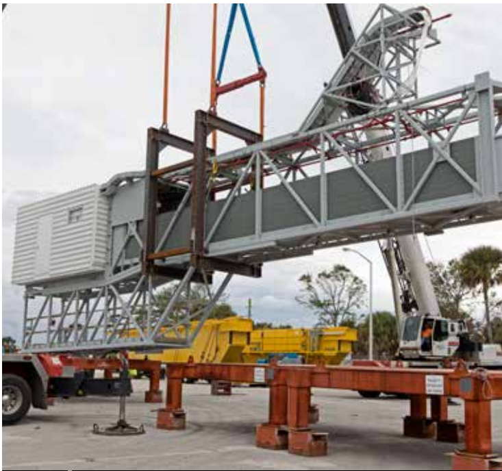
22 Crew Access Arm for Space Launch System Arrives at Kennedy
