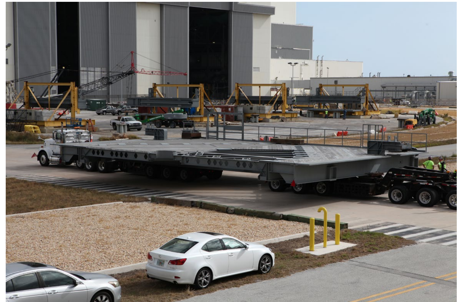
A heavy load transport truck from Tillett Heavy Hauling in Titusville, Florida, arrives at the Vehicle Assembly Building (VAB) at Kennedy Space Center, carrying the first half of the A-level work platforms, A north, for the agency's Space Launch System (SLS) rocket. The A-level platforms are the topmost platforms for High Bay 3 in the Vehicle Assembly Building (VAB). The platform will be delivered to the VAB staging area in the west parking lot. The Ground Systems Development and Operations Program is overseeing upgrades and modifications to High Bay 3 to support processing of the SLS and Orion spacecraft. A total of 10 levels of new platforms, 20 platform halves altogether, will surround the SLS rocket and Orion spacecraft and provide access for testing and processing. Photo credit: NASA/Ben Smegelsky
