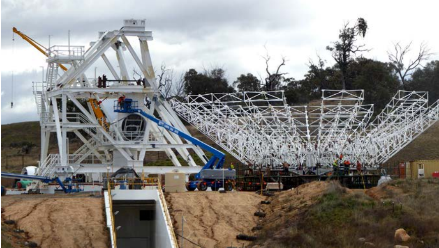
DSS-36 (34 meter Beam Wave Guide) under construction in Canberra, Australia
