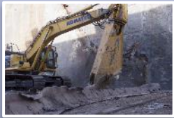
Completion of Pad 39B Flame Trench & Flame Deflector Construction
