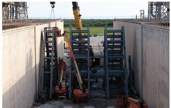
Cranes lower large segments of the support hardware for a new flame deflector into place in the flame trench July 21, 2017, at Launch Pad 39B at NASA's Kennedy Space Center in Florida. The new flame deflector will be positioned about six feet south of the shuttle-era flame deflector's position. During liftoff of NASA's Space Launch System, the rocket's flame and energy will be diverted to the north side of the flame trench. Photo credit: NASA/Kim Shiflett
