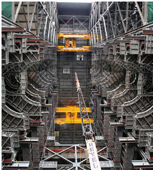
High up in the Vehicle Assembly Building (VAB) at NASA's Kennedy Space Center in Florida, an overhead crane lowered the final work platform, A north, into place for installation in High Bay 3 on Jan. 12, 2017. The installation of the final topmost level completes the 10 levels of work platforms, 20 platform halves altogether, that will surround NASA's Space Launch System (SLS) rocket and the Orion spacecraft and allow access during processing for missions, including the first uncrewed flight test of Orion atop the SLS rocket in 2018. Photo credit: NASA/Frank Michaux
