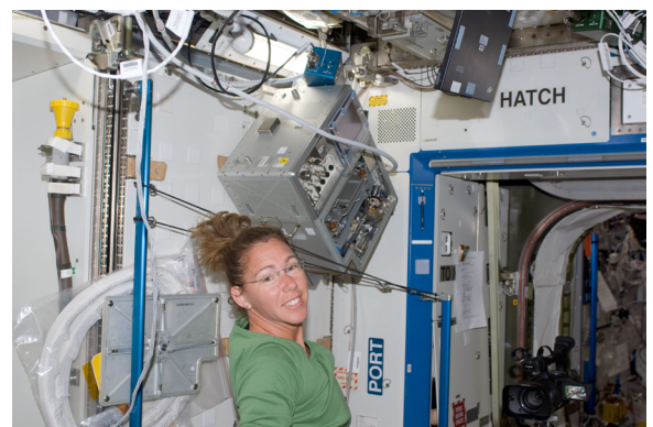
An astronaut installs a total organic carbon analyzer in the U.S. lab of the ISS
