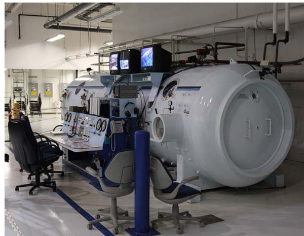
Figure 2: Hyperbaric chamber located at the NBL used to treat diving-related decompression illness
