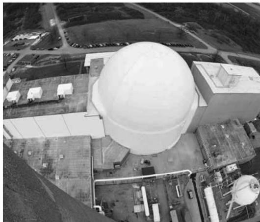
**The Space Power Facility is the world's largest vacuum chamber, 100 ft. in diameter by 122 ft. high, in which large space-bound hardware can be tested by simulating environmental conditions encountered in space. In support of NASA's diverse missions, Space Power Facility test programs have included high-energy experiments, rocket-fairing separation tests, Mars Lander system tests, deployable Solar Sail tests and ISS hardware tests.**
