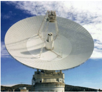
Figure 3. One of NASA's Deep Space Network antennae. This 70-meter (230 feet) antenna is from one of three DSN facilities that are positioned around the globe approximately 120 degrees from each other so that as Earth rotates at least one antenna is always “visible” from space.. (Image courtesy: NASA/JPL)
