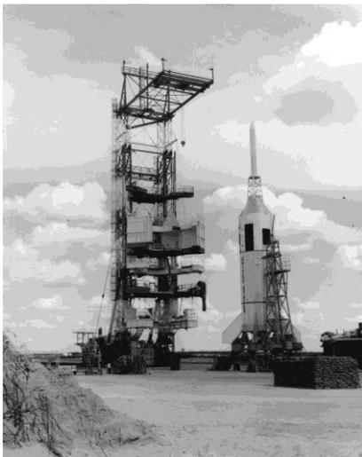
For the Apollo program, NASA developed an escape system for the crew if there was a failure during launch. From 1963 to 1966 a series of tests was conducted using a Little Joe II rocket to simulate the Saturn rocket. It was capable of carrying the boilerplate Apollo capsule to an altitude of 31,000 feet at speeds similar to an actual launch.
