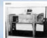
The Wind Tunnel: The Wrights tested small model wings in a wind tunnel that enabled them to calculate the wing shape and size that would be required to lift them into the air.
