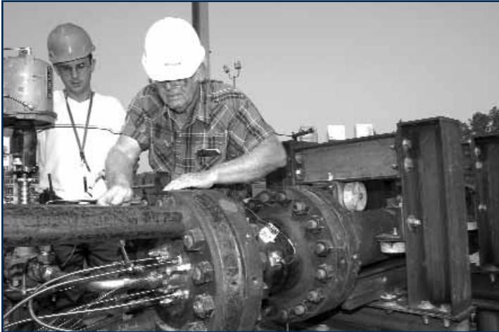
Jared Grover (left), a NASA test conductor, watches as R.B. Shaw, a mechanical technician, works on a gaseous oxygen line prior to the test-firing of a paraffin-fueled rocket motor.
