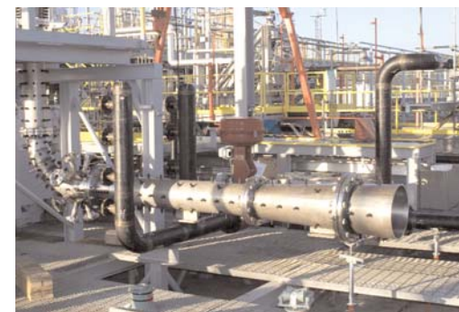
A-3 TEST STAND MILESTONES – At top, NASA officials event Aug. 23 for the A-3 Test Stand at Stennis Space Center. Administrator for Exploration Systems Doug Cooke, Pratt & Whitney Director Richard Gilbrech, NASA Associate Administrator Administrator Shana Dale, Mississippi Gov. Haley Barbour, Stennis Deputy Director Gene Goldman and A-3 Project Manager version of A-3's exhaust diffuser in Stennis' E Complex here.
