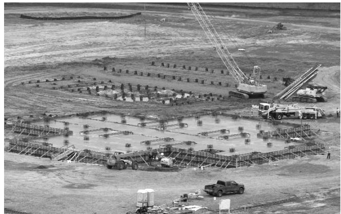
**FINISHED PRODUCT** – With concrete in place Dec. 9, the 160-foot-by-160-foot A-3 base takes shape. The foundation remained under plastic cover for about seven days, and will be allowed to cure undisturbed over the next several weeks. The mix of the material is designed to bear a load of 4,000 pounds per square inch when hardened.
