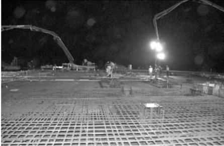
**STRONG FOOTING** – A field of steel rebar forms the frame for the concrete that will become the base of the A-3 Test Stand at Stennis Space Center. The weight of all the steel in A-3's foundation equals more than 1.5 million pounds.
