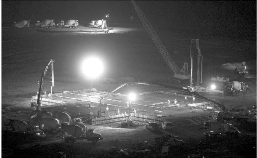
**LIGHTING THE WAY** – Floodlamps illuminate the site of Stennis Space Center's future A-3 Test Stand as concrete trucks jockey for position to deliver their product. Over a 14-hour period beginning at 6 p.m. Dec. 8, more than 400 trucks delivered 3,365 cubic yards of concrete for the stand's foundation. The task was scheduled at night to ensure an uninterrupted traffic flow on local and on-site roads.
