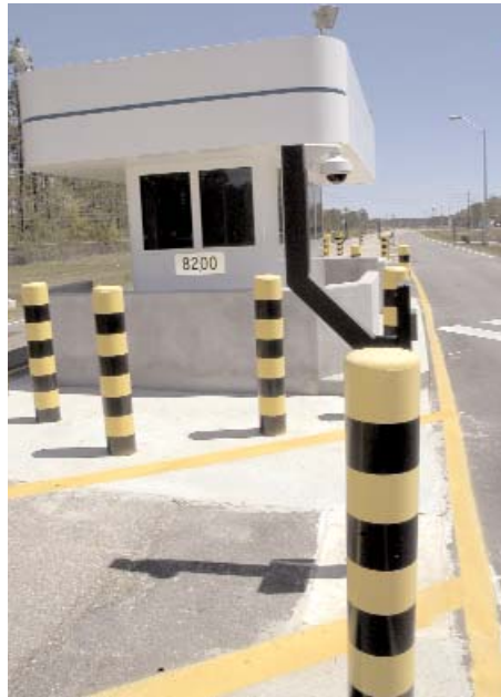
Saturn Drive gate to test complex
