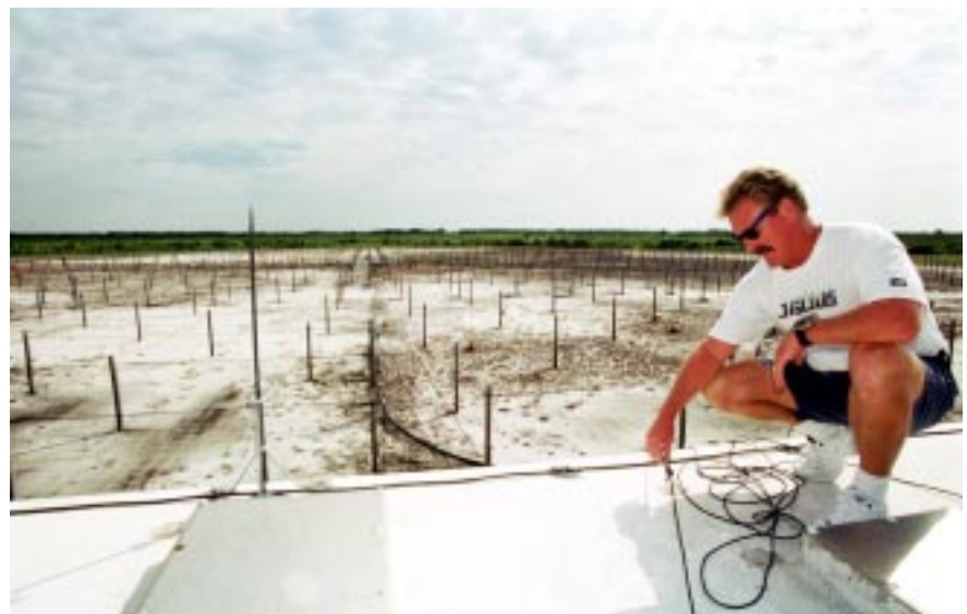
Eric Fetzer, an RF technician with CTI, checks a a cable at the Doppler radar wind profiler station, which is located near the Shuttle Landing Facility.
