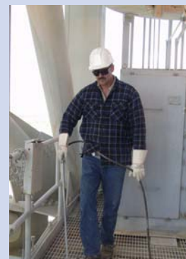
At left, Rick Mako, Joe Rosenbaum and Paul Dinicola modify a bracket for the External Tank vent arm. Below, Alan Baleyko cleans off rust and oxidation from the structure of Pad B during preparation for the STS-110 Mission launch of Atlantis.
