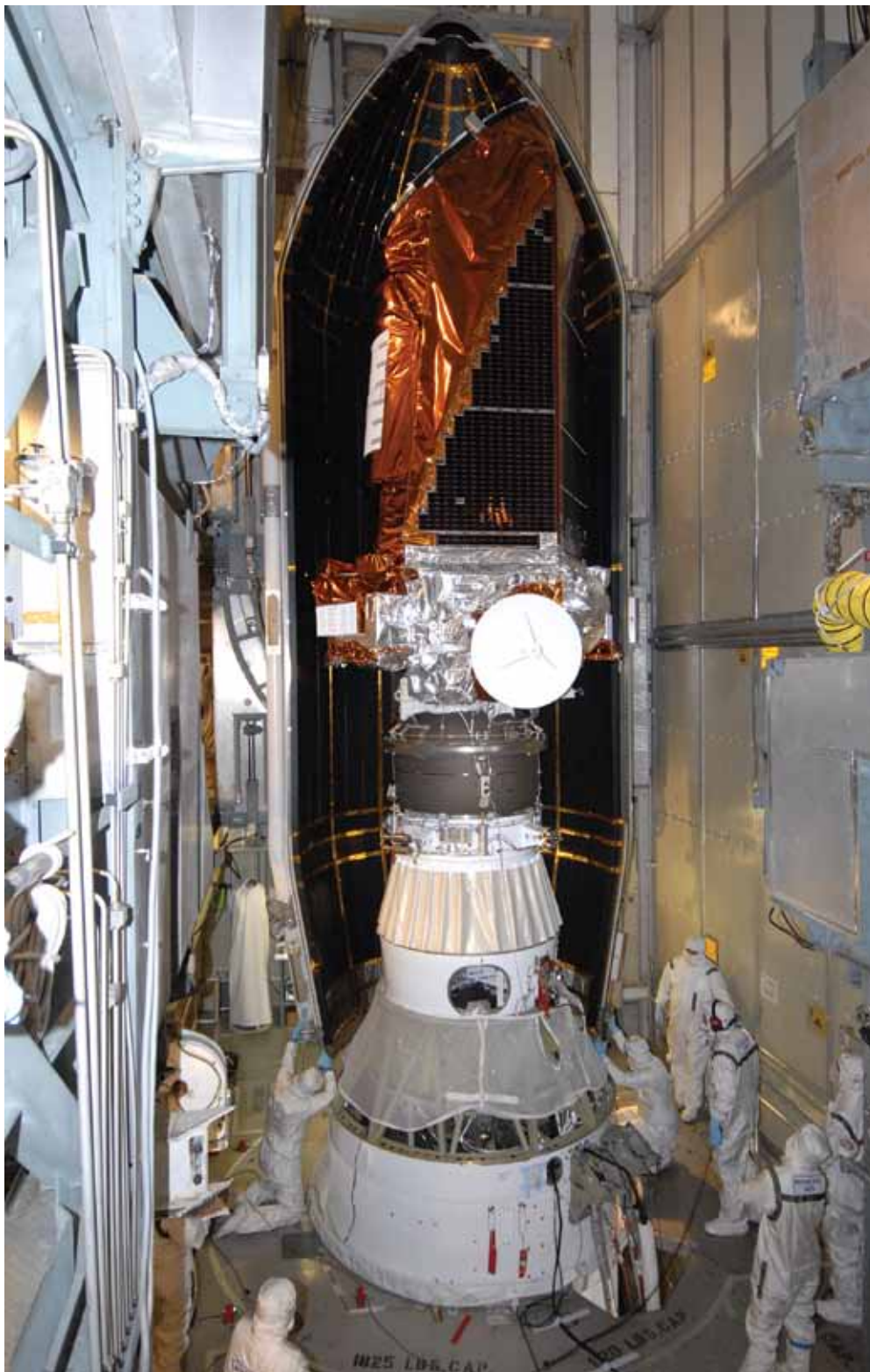
On Launch Pad 17-B at Cape Canaveral Air Force Station in Florida, the first half of the fairing moves into place around NASA's Kepler spacecraft, atop the United Launch Alliance Delta II rocket. Kepler is designed to survey more than 100,000 stars in our galaxy to determine the number of sun-like stars that have Earth-size and larger planets.
