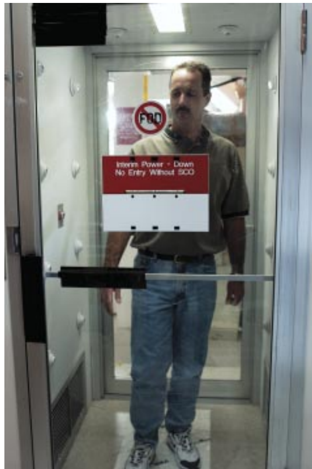
A KSC employee uses a clean-air shower before entering a clean room. Streams of pressurized air directed at the occupant from nozzles in the chamber's ceiling and walls are designed to dislodge particulate matter from hair, clothing and shoes. An adhesive mat on the floor captures soil from shoe soles.
