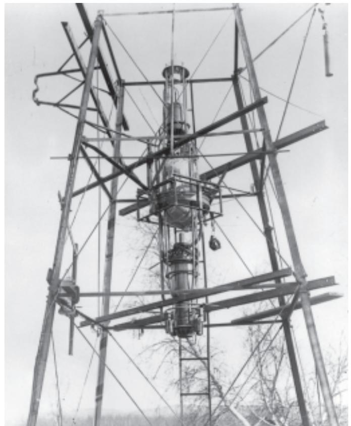
Setup for Dr. Goddard's test of April 20, 1927, with parachute attachment and turntable for launching, at Auburn, Massachusetts. *Photo courtesy of Mrs. Robert H. Goddard.*
