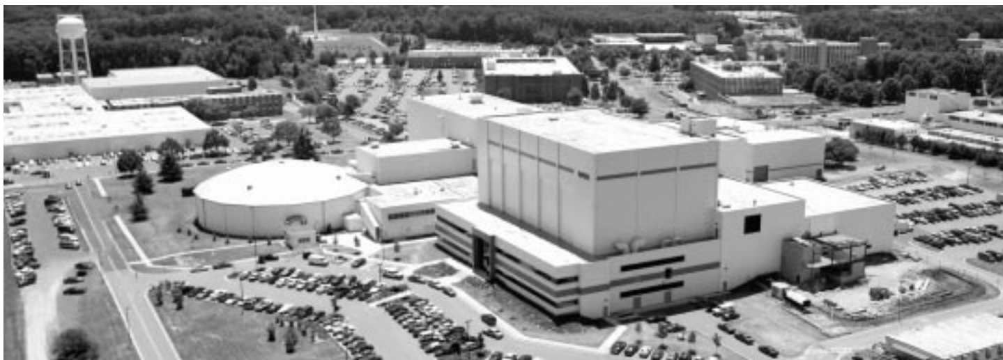
Key facilities shown in the foreground of this aerial view of Goddard include the Spacecraft Systems Development and Integration Facility, which contains one of the world's largest "clean rooms"; the Spacecraft Test and Integration Facility, which contains thermal-vacuum chambers, a vibration platform, and an acoustic test chamber; and the High Capacity Centrifuge (circular building), which houses a rotary accelerator capable of rotating 5,000-lb payloads at up to 30-times Earth's normal gravity.
