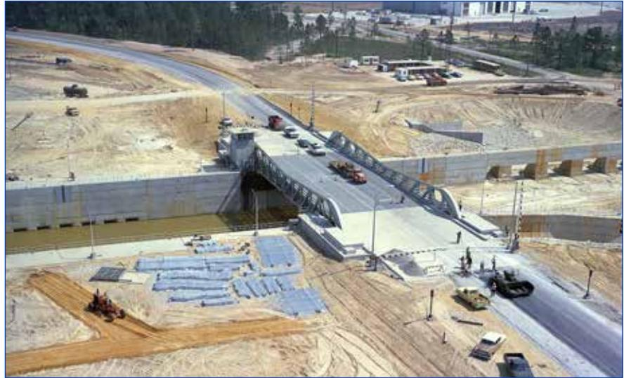
A 1965 photo shows final construction of the bascule bridge still in use at Stennis Space Center.
