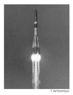
A rare picture of the 8K78 threestage rocket, which launched a series of Soviet lunar and deep space probes in the early 1960s. This particular image shows the launch of a 2MVtype space probe.
