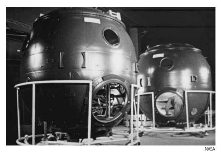
Soyuz orbital modules being assembled at the Factory for Experimental Machine Building (ZEM) next to Korolev's design bureau.
