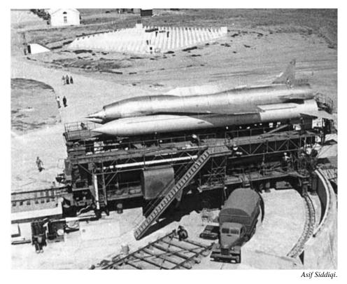
The Burya missile (with the internal designation '350') was the first Soviet intercontinental cruise missile. Developed as an alternative to the R-7 intercontinental ballistic missile, the Burya was launched nearly 20 times between 1957 and 1960 before being cancelled.
