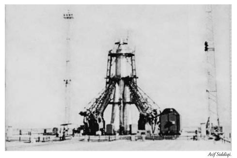
This photo shows Sputnik-3 (Object D) on the launch pad prior to launch in 1958. This satellite used a one-off variant of the R-7 ICBM known as the 8A91. Note the unusual tip of the payload fairing.
